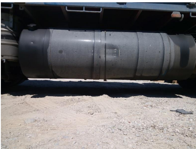
Picture 15: Strap the sensor before the glue work time expires. Use 16mm steel strapping tape. This picture is taken with plastic tape. You can see the sensor at the bottom of the tank.
