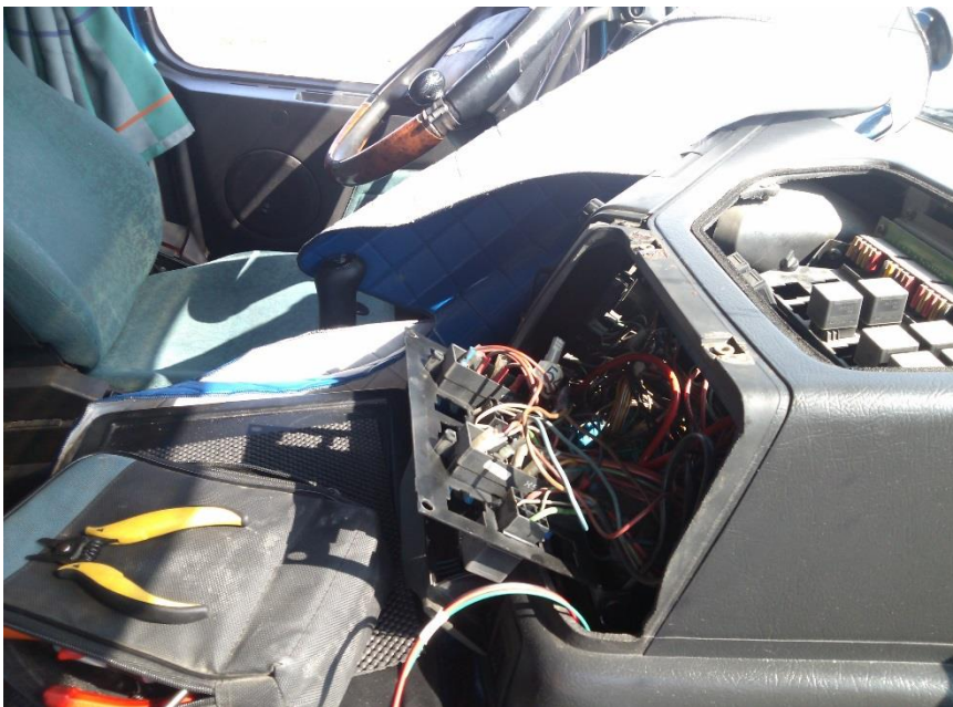
Picture 10: connecting power and ground
